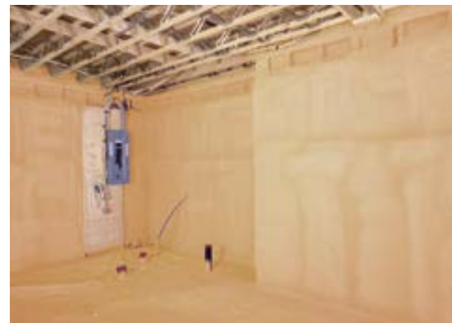
WALLTITE® applied on basement walls and under slab
