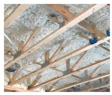
ENERTITE® Max is a low-density open-cell SPF insulation, formulated for high-yield application performance while meeting GREENGUARD Gold standards. It is ideal for insulation and air sealing applications in residential and commercial construction. ENERTITE Max provides contractors with improved yield, consistent thermal values, and superior overhead application performance.
