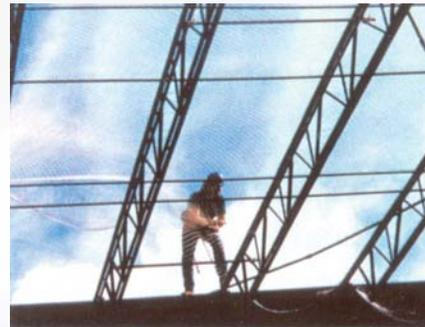
Sky-Web II® is a made-to-order product that arrives at the job site with all of the instructions and required hardware necessary to complete the installation. The system consists of a 2 3/4" x 2 3/4" knotted nylon mesh that can accommodate every building configuration,
